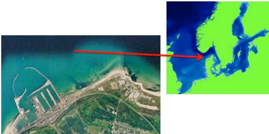
Fig. 1 Location of the Port of Hanstholm on the northwestern coast of Denmark
